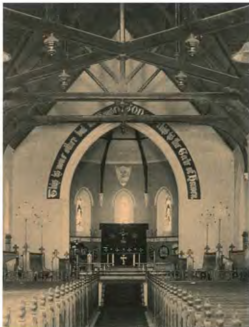
Interior pre 1890, showing stencilling
